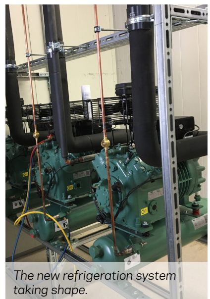
Lines and pipework installed on the deep-freeze cold store
