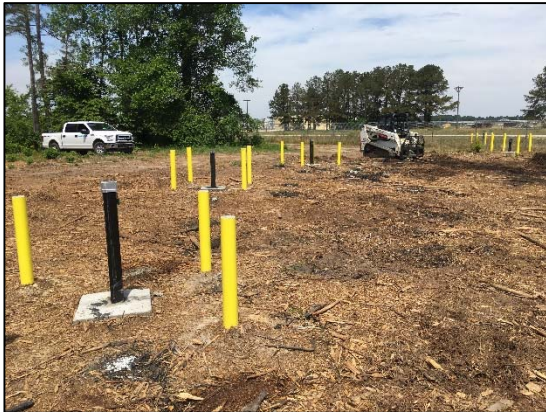
Photo 21: Perched Zone after completing injections. MWs 34-36 pictured.
