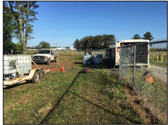
Photo 2: Staging area for RRS equipment, water, and product.
