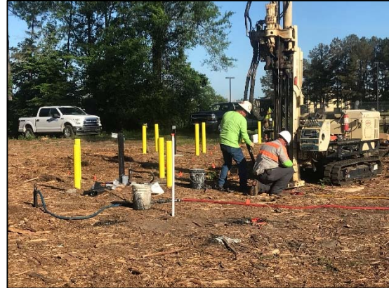
Photo 20: Injections in progress in the Perched Zone Area.
