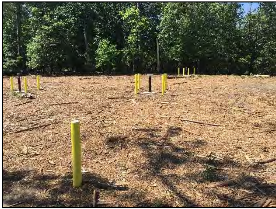
Photo 1: Perched Zone Pilot Study prior to the PlumeStop application. MW-35 pictured in center.
