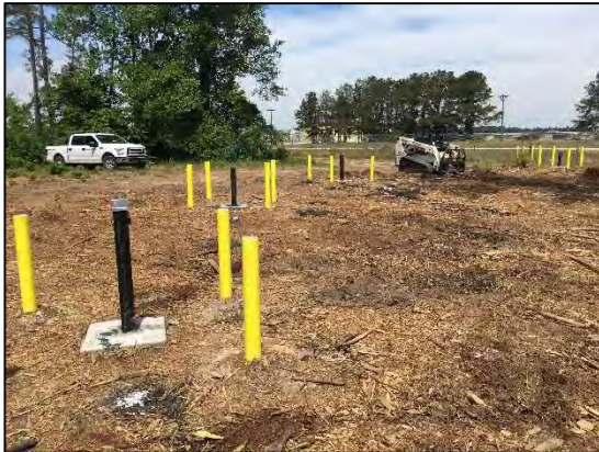
Photo 21: Perched Zone after completing injections. MWs 34-36 pictured.
